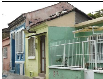
Figure 9: The colorful buildings at the grid urban pattern
